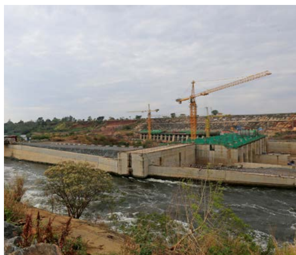
Karuma Hydro Dam, Uganda
